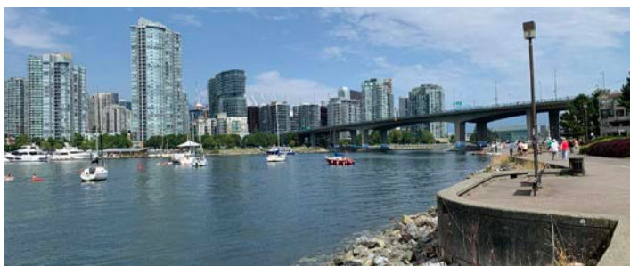
Vancouver Seawall along False Creek looking towards Cambie Bridge - Merv Mascarenhas
